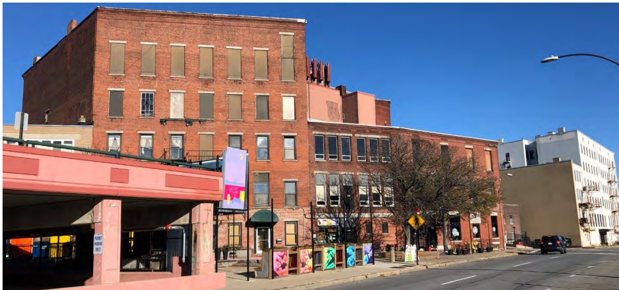
View looking east to Mill Street on Boulder Drive
